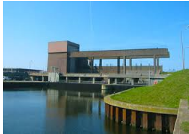
Europe's largest pumping station
