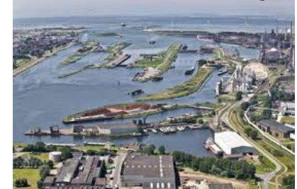
Eight locks, including IJmuiden Locks Complex
